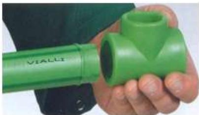
**3.) Within the allowed time interval, connect the pipe and Fitting (do not twist)**
